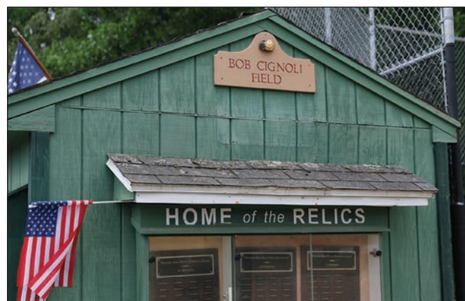
The field house near the Relics softball fields.
